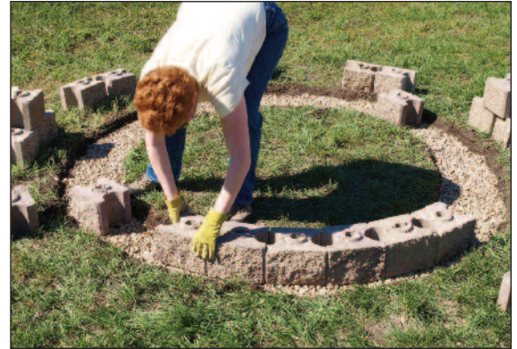
Install First Course
