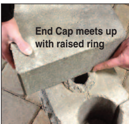
Flip the AB York block over below end cap
