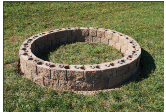
Install Second Course
