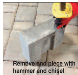
Flip the AB York block over below end cap
