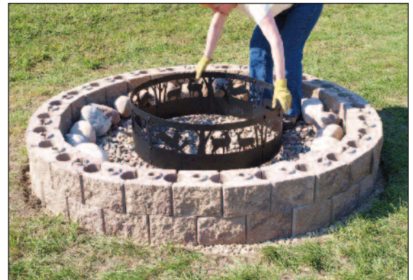
Install Decorative Rock and Fire Ring
